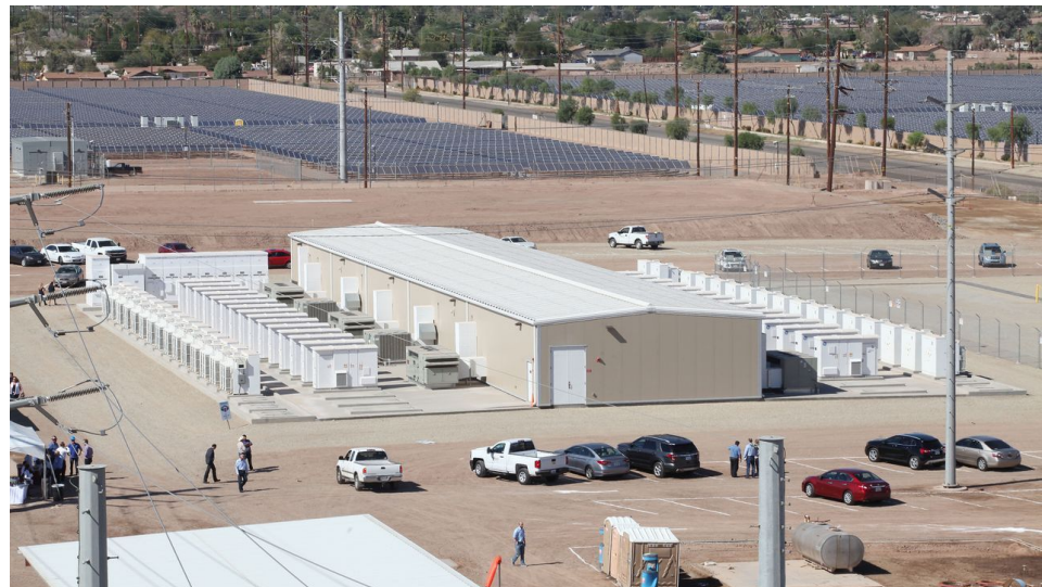
Imperial Irrigation District's Battery Energy Storage System
