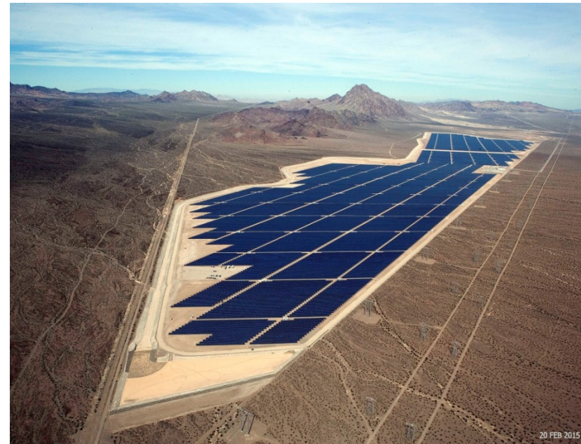
Copper Mountain Solar Project
