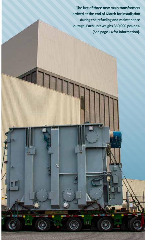
The last of three new main transformers arrived at the end of March for installation during the refueling and maintenance outage. Each unit weighs 350,000 pounds. (See page 14 for information).
