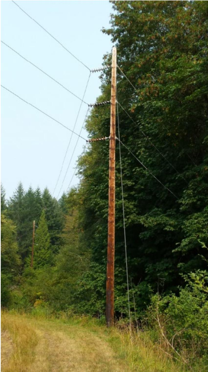
**Figure 3. Corner pole with insulators in a vertical row.**
