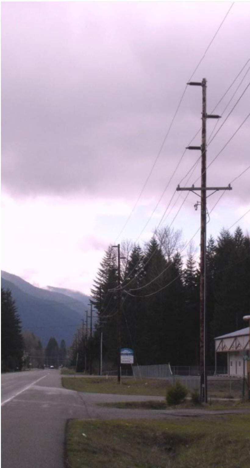
**Figure 5. Vertical conductor design used along Highway 12.**
