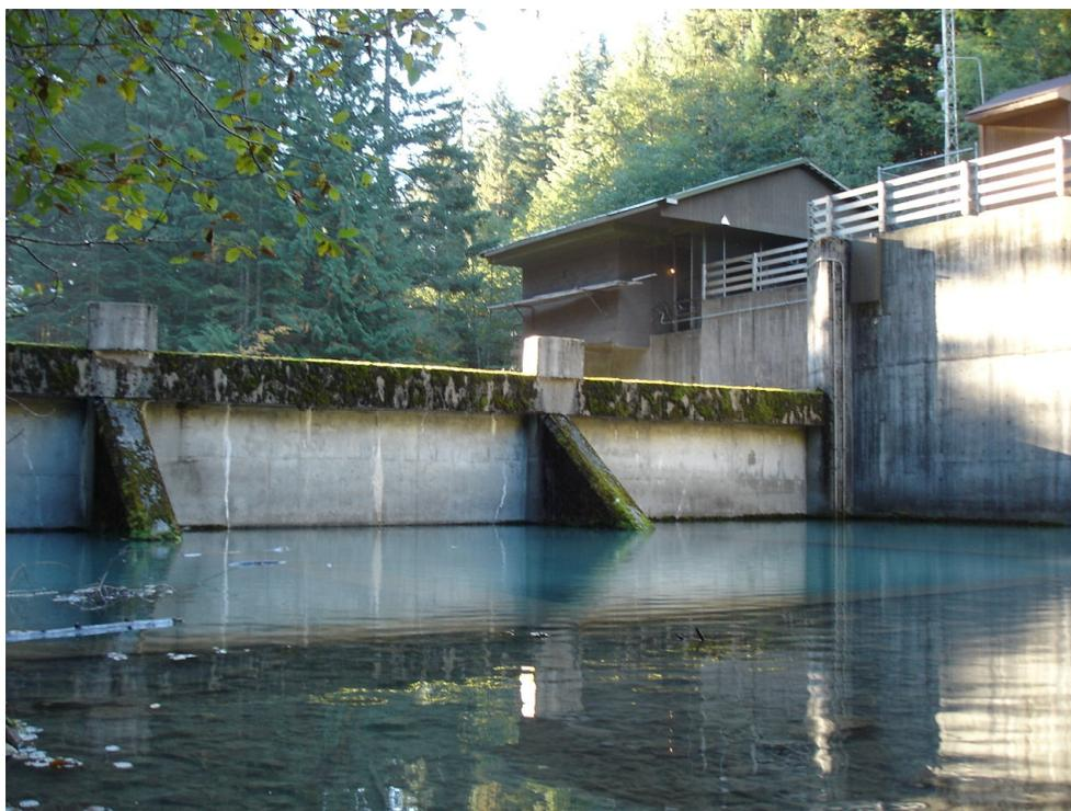
Figure 1-1. Packwood Lake Hydroelectric Project Drop Structure
