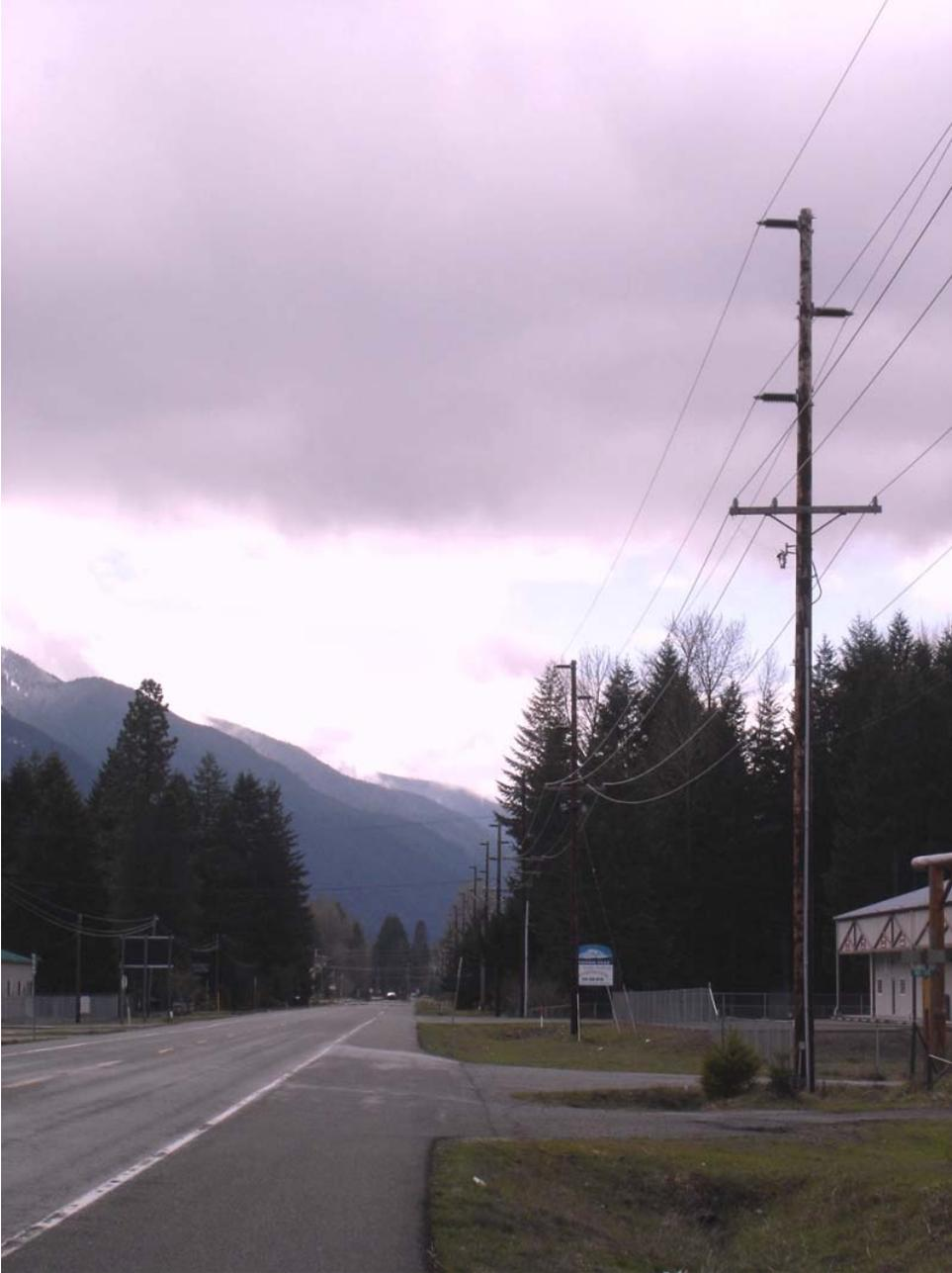
**Figure 4. Vertical conductor design used along Highway 12.**
