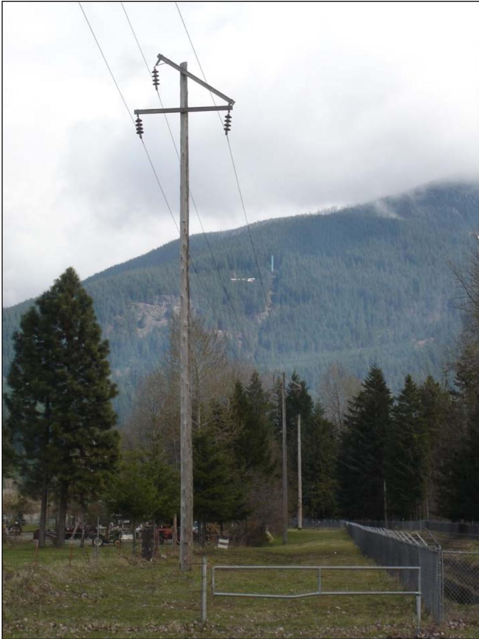
**Figure 2. Transmission line adjacent to project tailrace canal, showing wishbone conductor configuration.**
