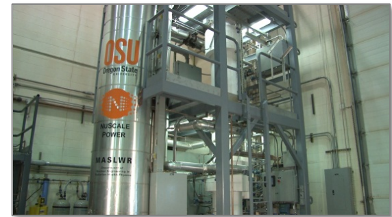
One-third scale Test Facility
