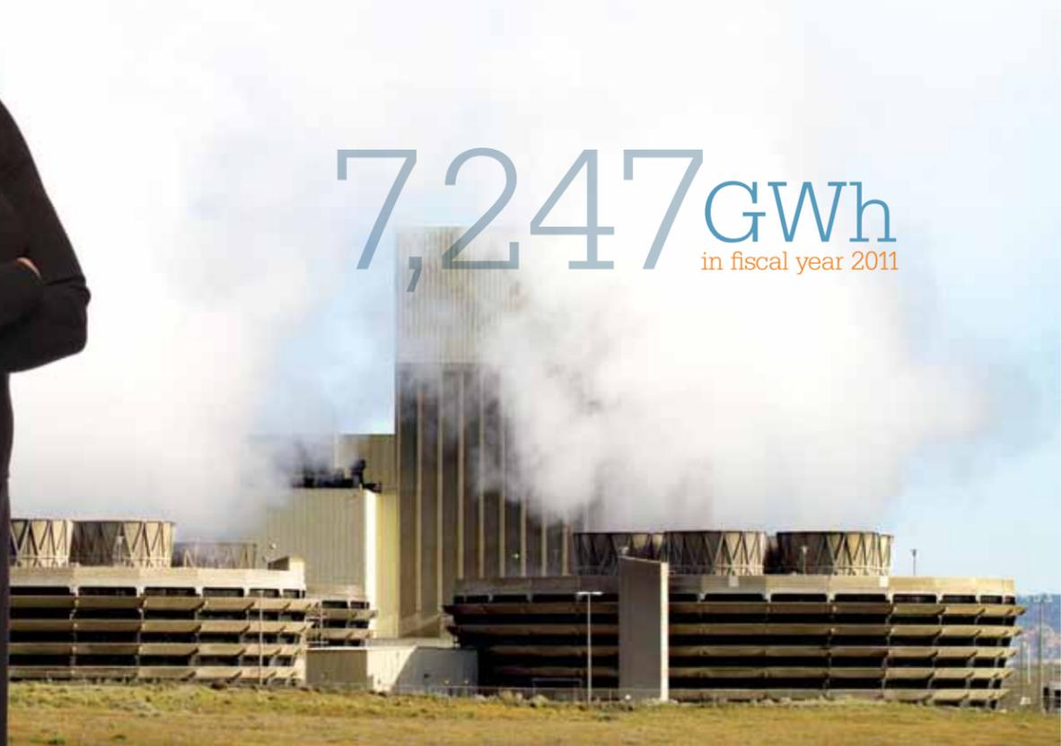
Columbia Generating Station is a boiling water reactor, or BWR. Columbia produces 1,150-megawatts of electricity, enough energy to power more than a million homes. Columbia began commercial operation in December 1984.
