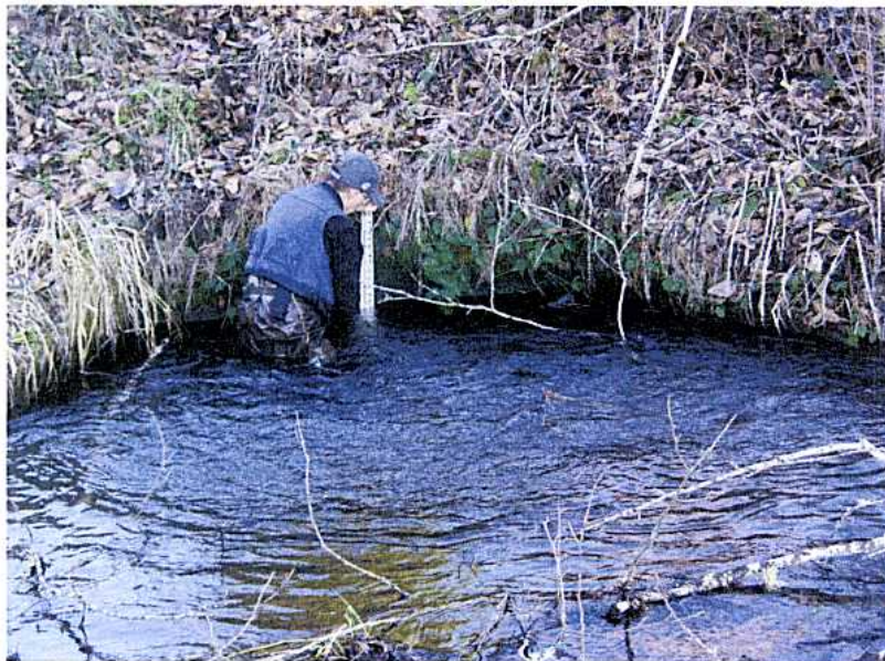
Photo 6. Downstream entrance of culvert on Snyder Creek, below tailrace.
