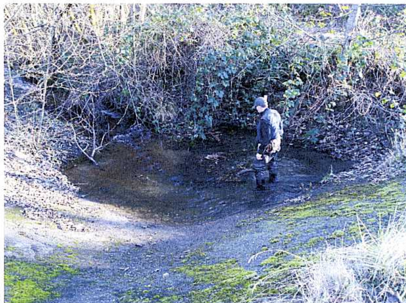
Photo 4. Drain and stilling well on Snyder Creek, upstream side of tailrace.
